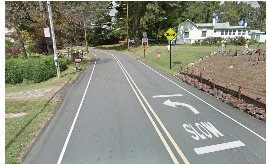
Examples of Speed Signs and Markings: Speed Feedback Signs (Left Side of Road), Slow Warning Sign (Right Side of Road), and Slow Pavement Markings (in Right Lane).
