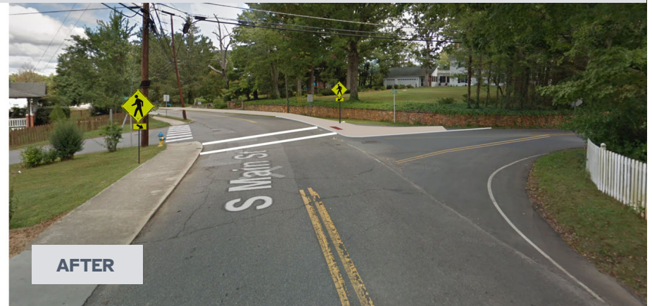
Hillside at South Main Street Short Term Application: Reduce radius and implement Pedestrian Crossing with signs and markings. Possible long term implementation option with curb extensions and ADA ramps.
