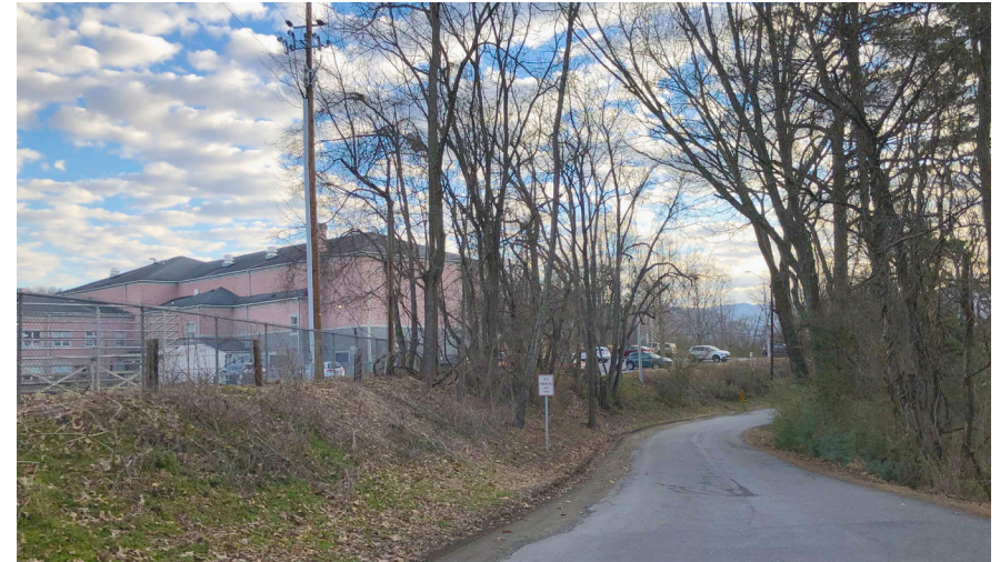
Given the Roadway Constraints, this Project May Be Best Aligned on the School Property Near the Fence; Close Coordination is Necessary During Project Development.
