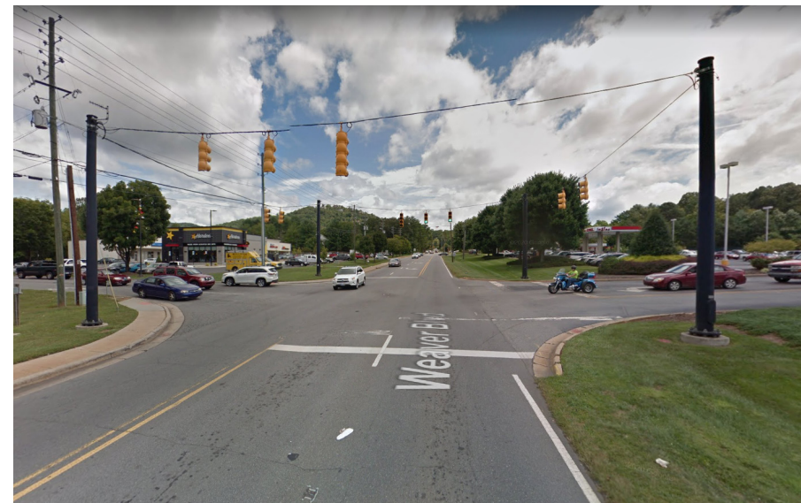
Weaver Boulevard at Ingles Signal: Missing Crosswalks, Pedestrian Signals and Curb Ramps.
