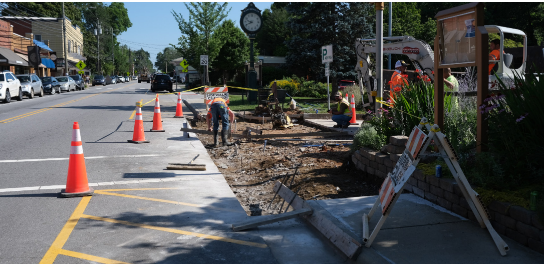
Image 4. Curb Ramp Upgrades Being Led by NCDOT on Main Street in 2021.
