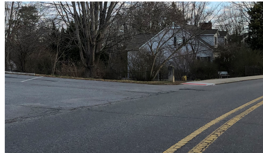
Sidewalk Gap at the Faculty/Staff Parking Area of the Elementary School.
