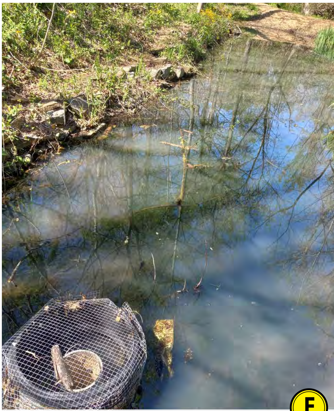
OUTLET AT NORTH POND
