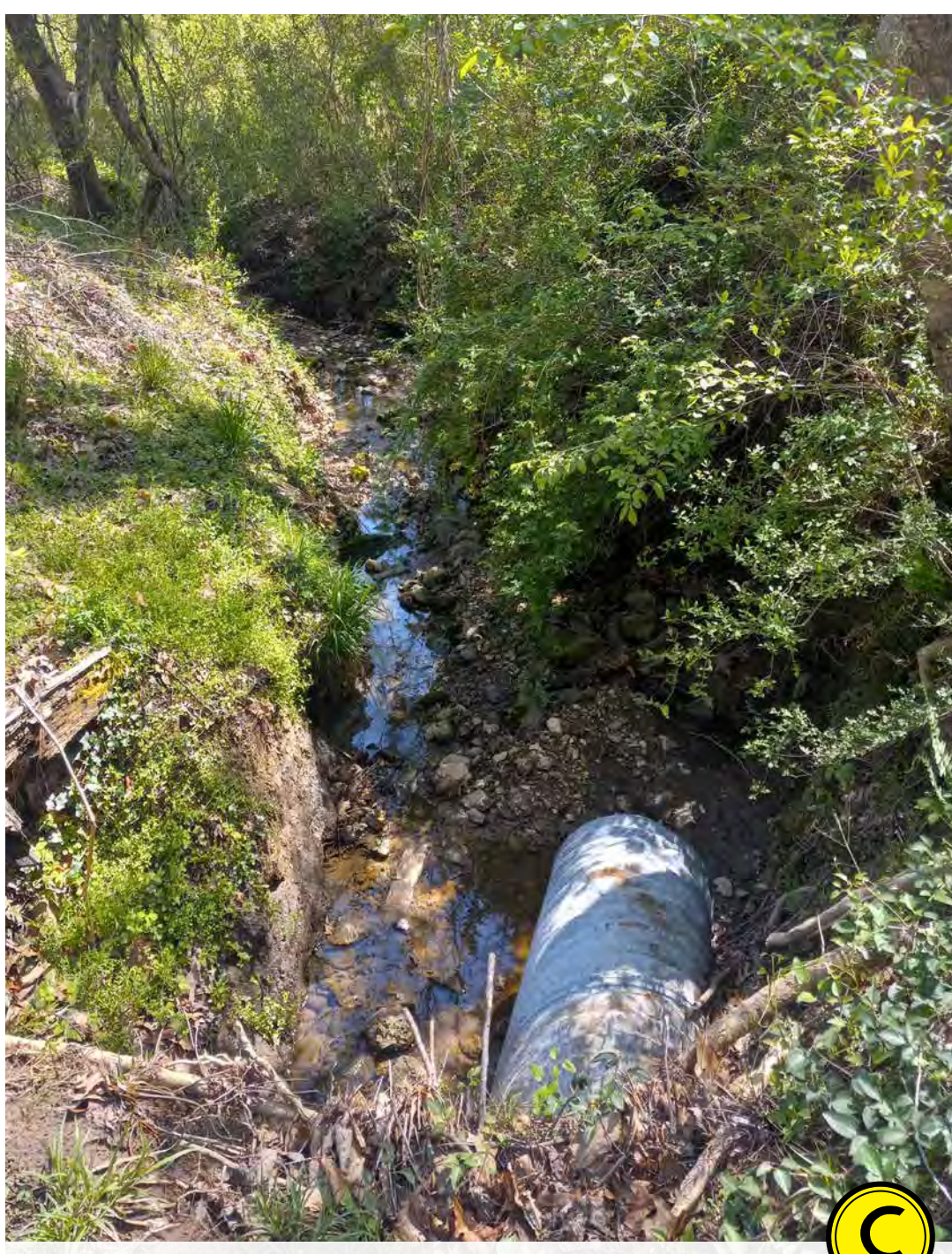
CULVERT ALONG CREEK
