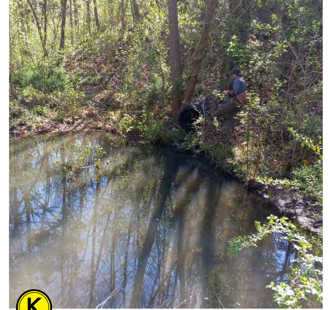
SOUTH STORMWATER POND
