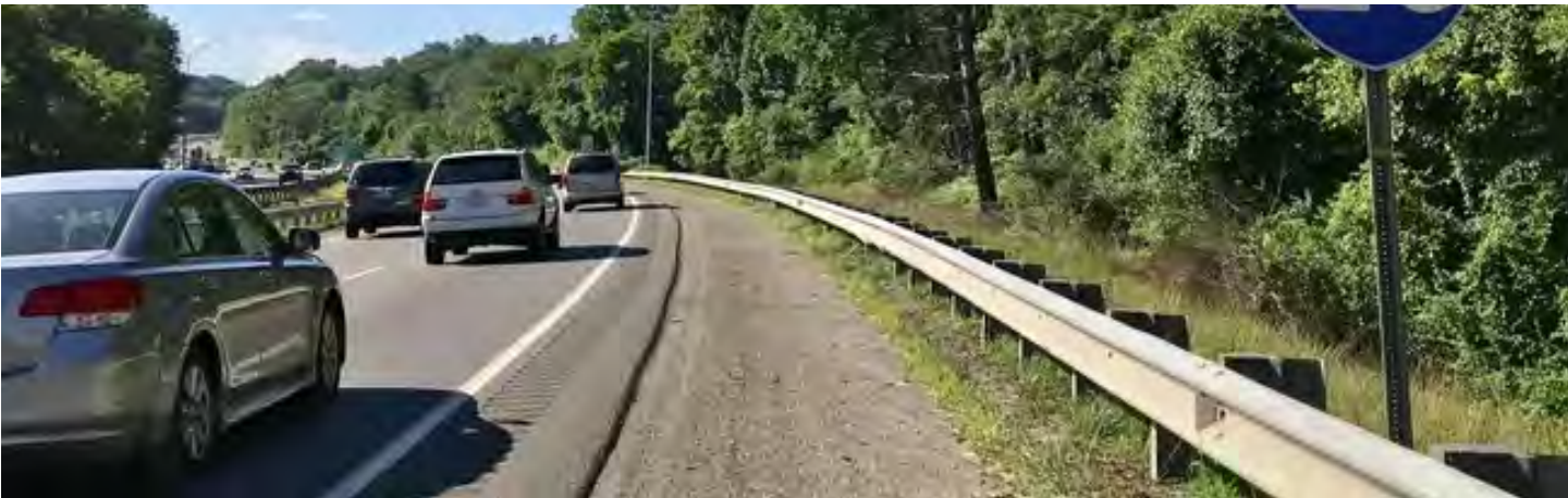
A gravel shoulder, guardrail, and adjacent wooded area illustrate the physical space and context for a potential multi-use path paralleling the interstate.
