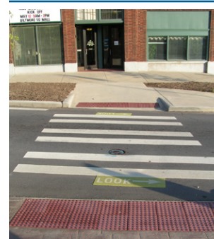
Connections to the greenway
