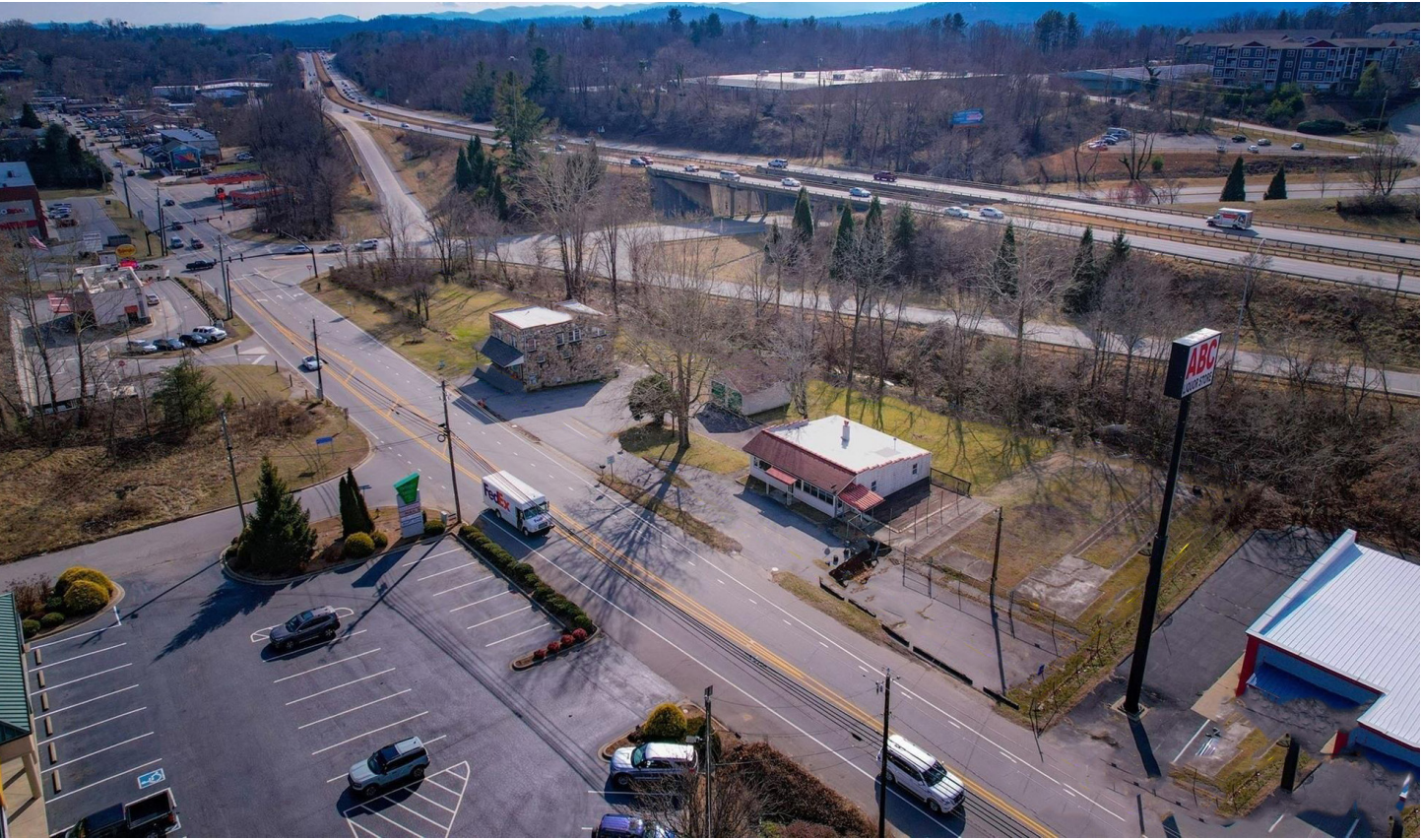
Commercial development, frequent driveways, and adjacent parking areas characterize this corridor and influence access, safety, and feasibility considerations for a potential sidepath.
