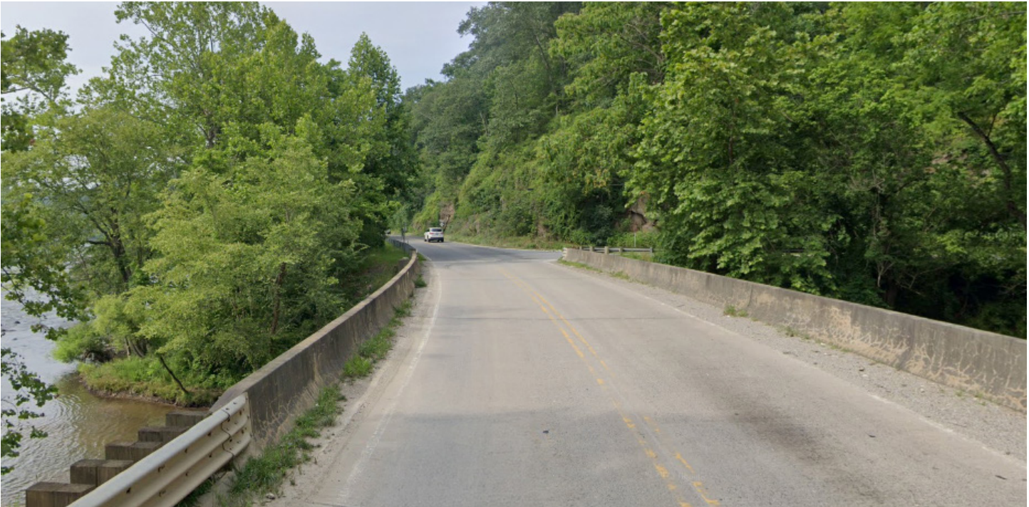
Image 14. Bridge Over Reems Creek
