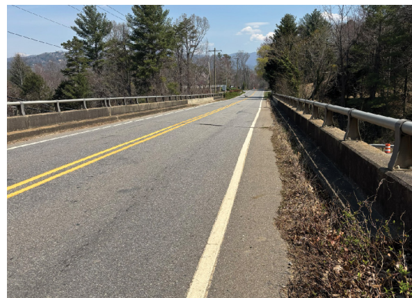
Segment 20: Aiken Road Bridge over I-26.
