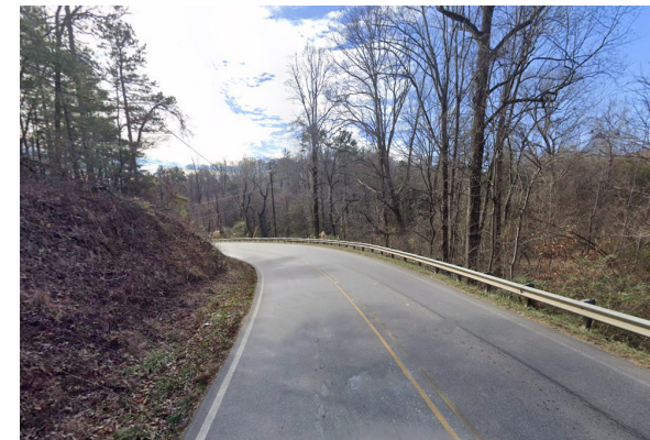
Segment 12: Further north along Riverside Drive includes significant challenges for constructing a multi-use sidepath including steep slopes on both sides of the roadway.
