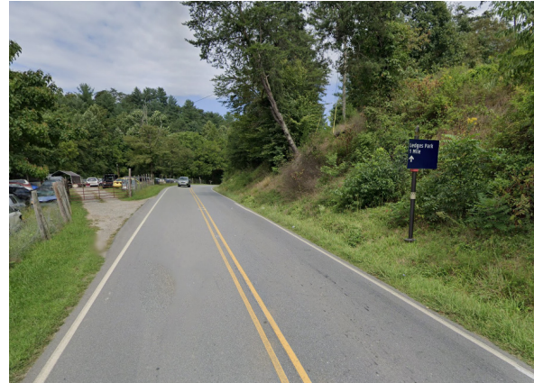
Segments 13 + 14: Old Marshall Highway is a two lane road with longitudinal slopes of up to 8%, making this a challenge to developing a sidepath.
