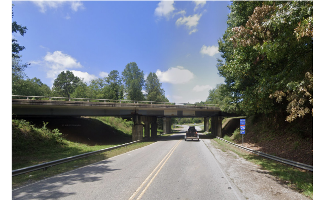
Segment 18: New Stock Road under the interstate includes just over 11' between the edge of road to the guardrail.
