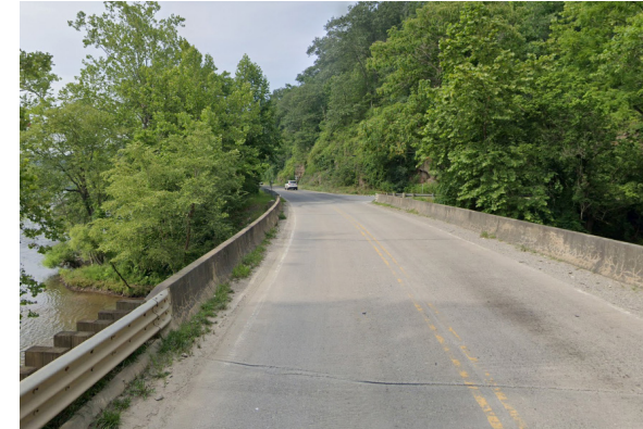
Segment 31: A constraint to a multi-use sidepath in the northern Riverside Drive is a vehicle bridge over Reems Creek with narrow shoulder widths.
