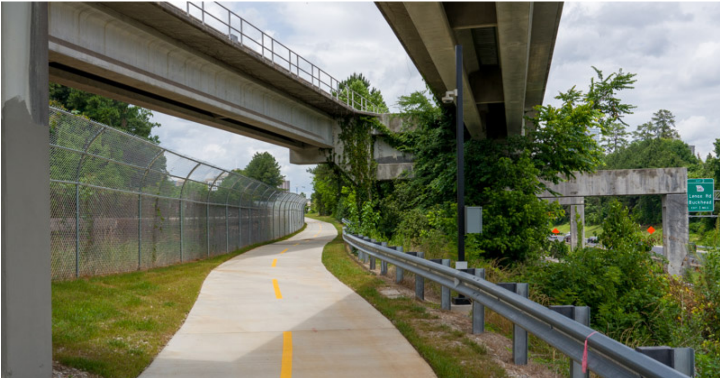
The PATH 400 trail navigates a complex urban highway environment with guardrails, fencing, and elevated structures, demonstrating how thoughtful design can balance safety, separation, and user experience.
