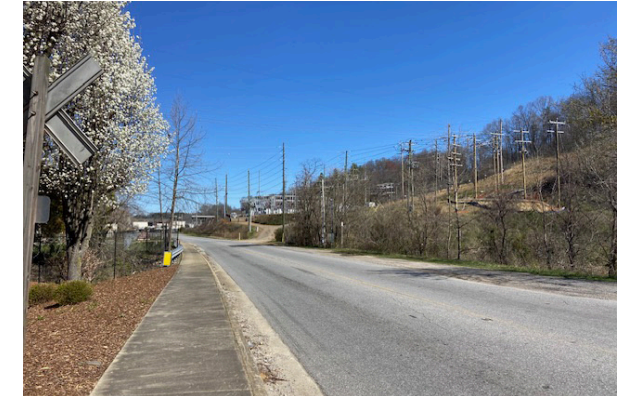
Segment 12: North of Municipal Sewer District on Riverside Drive includes a sidewalk on the river side and a significant slope of the opposite side.
