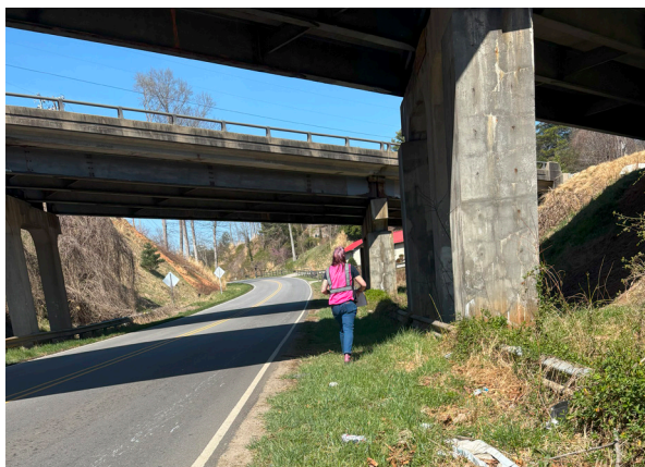
Segment 14: At I-26 overpass at Old Marshall Highway.
