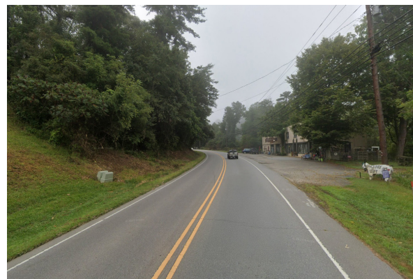
Segment 8 and 9: As Weaverville Road gets closer to Weaverville, the terrain gets more steep adjacent to the roadway.
