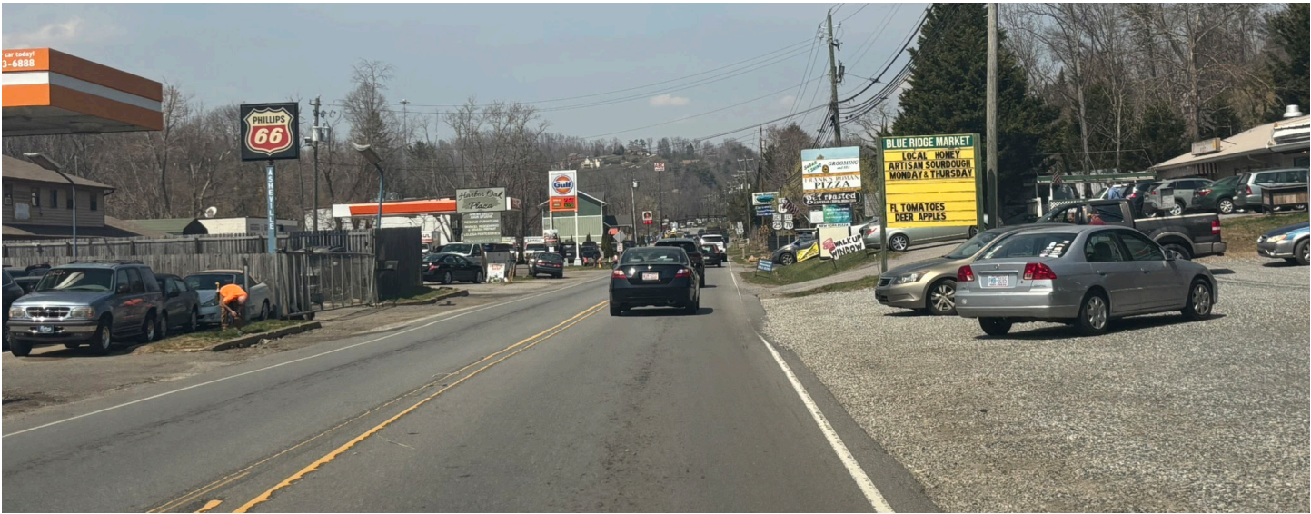
Weaverville Road serves as a key connection between Woodfin and Weaverville, with constrained right-of-way, adjacent commercial development, and numerous driveway and access points.
