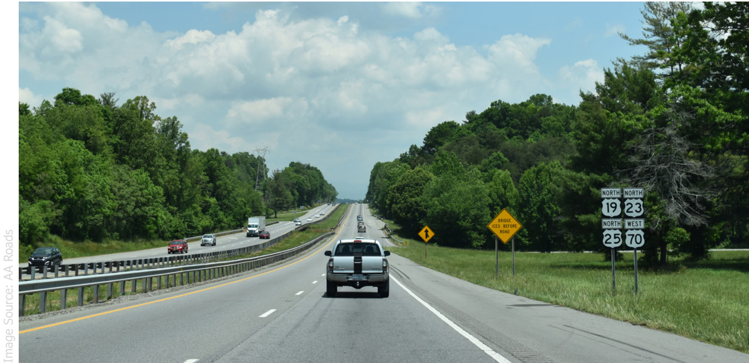
At the New Stock Road interchange, the northbound lanes of I-26 show the eastern edge of the corridor where a buffered multi-use path could be accommodated as part of Alternative A.
