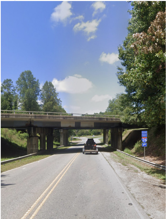
New Stock Road passing beneath I-26 represents a critical access point for Alternative A, allowing users to enter and exit the corridor and connect to nearby streets and destinations.
