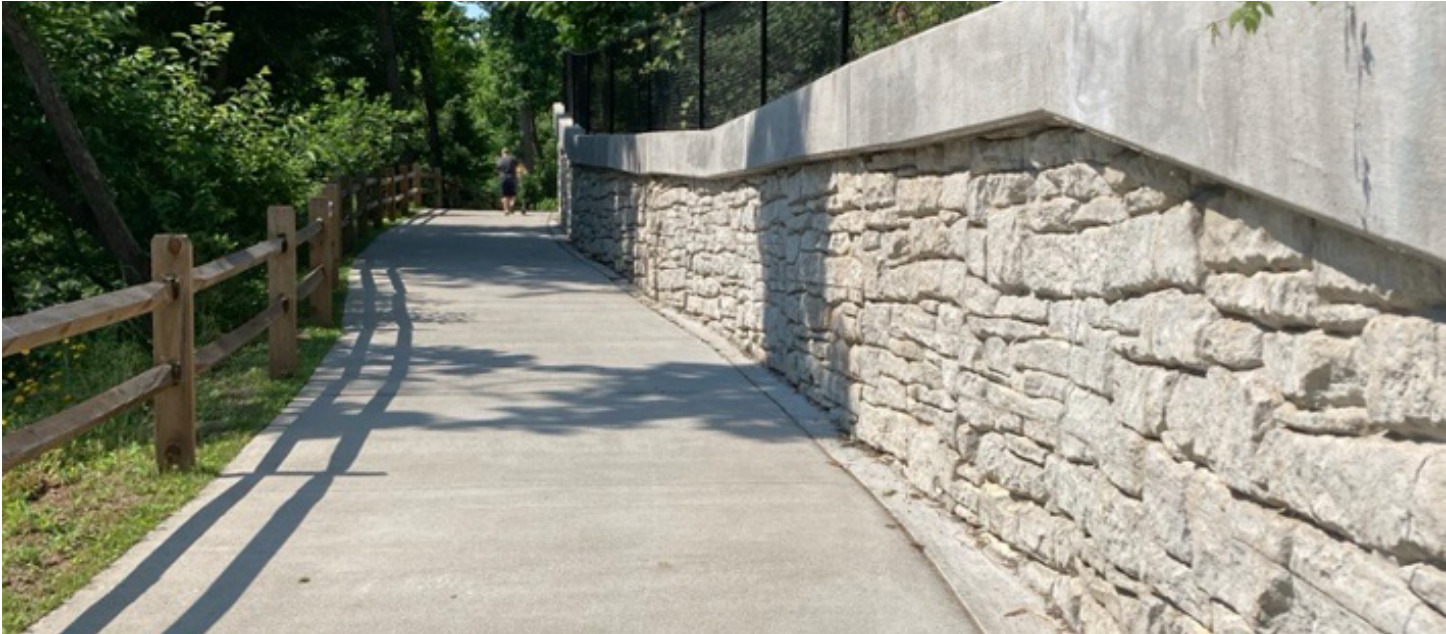
Image 44. Retaining Wall (French Broad River Greenway)
