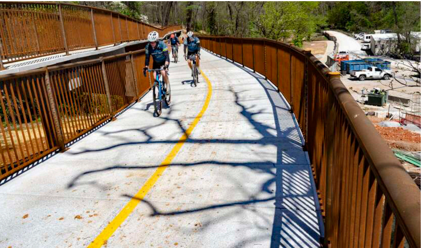
Image 45. Flyover Bridge (Razorback Greenway)
