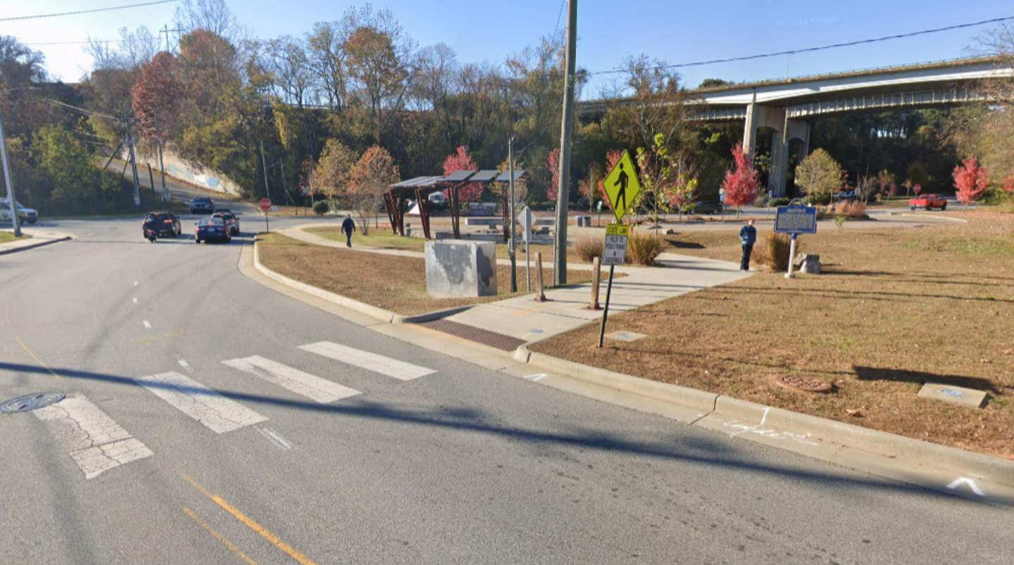
High-visibility striping, signage, and ADA-compliant ramps provide a safe and accessible connection between a trailhead and the French Broad River Greenway.
